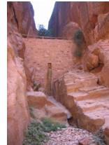
The Nabataeans were master engineers and urban planners. To prevent powerful winter rains and flash floods from entering the Siq, for example, the Nabataeans built dams wherever water might enter the canyon.
