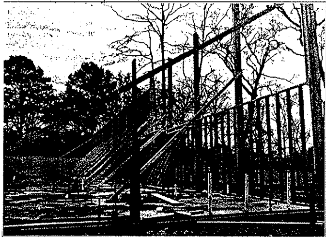
Construction is underway at church property on Lake Palestine
